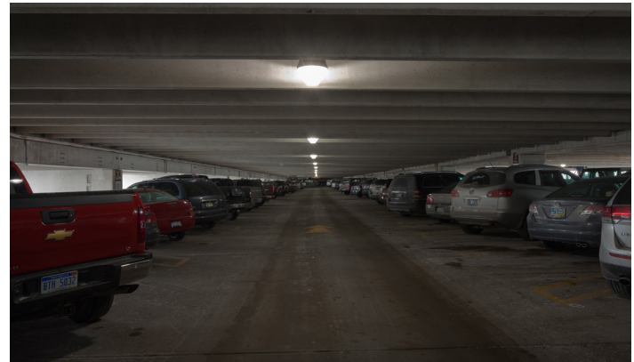
Before new lighting system
