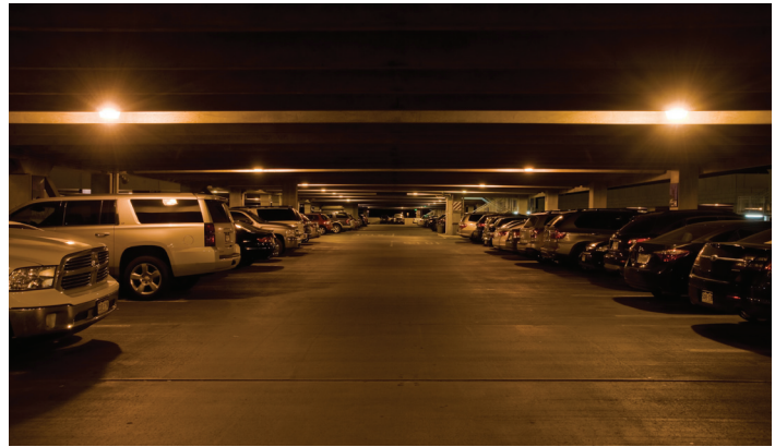
Before new lighting system
