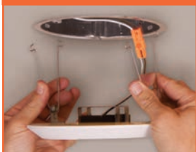
6-inch torsion spring position
