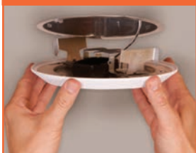
6-inch friction clip position
